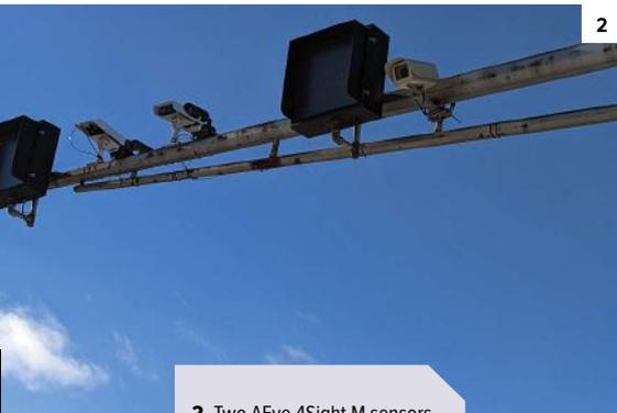
2. Two AEye 4Sight M sensors installed to monitor 1km of highway for AID systems
